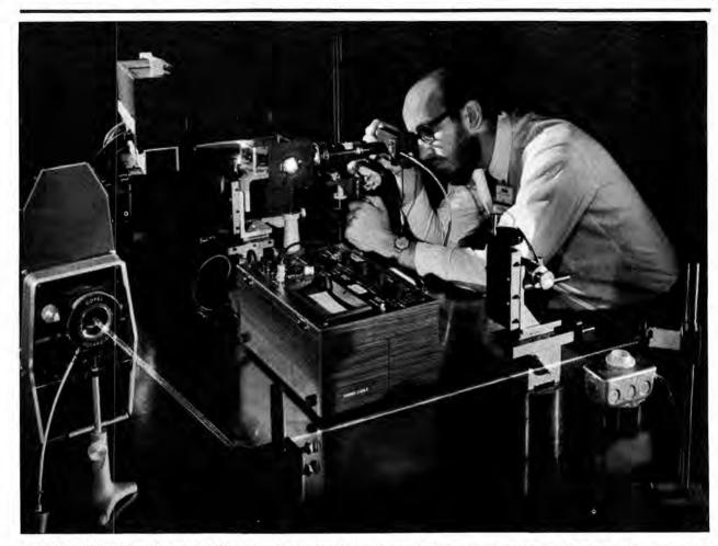
STRESS ANALYSIS OF A MATERIAL (in lucite container at end of microscope) is made by Wil Jorgenson of Experimental Mechanics Division 8122 using scattered light photoelasticity technique. The technique is effective for finding stress loads with complex geometric shapes in which dissimilar materials are used.
